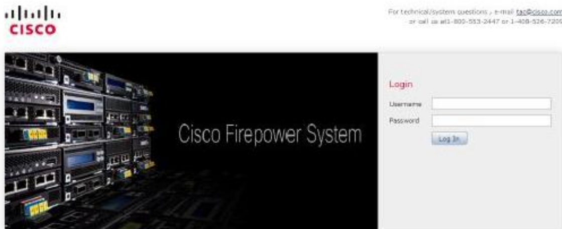
Fig CISCO Firepower System at ICS Server Room
