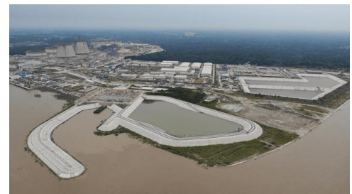
Picture: Water Intake Structure
