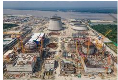
Picture: Birds Eye View of Rooppur NPP Project Site
