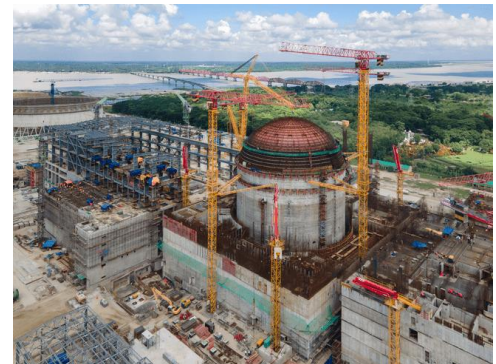
Picture: Reactor Building of Power Unit-2
