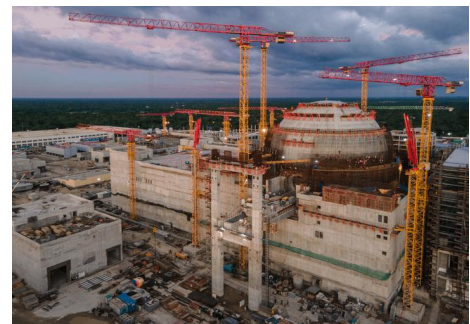
Picture: Reactor Building of Power Unit-1
